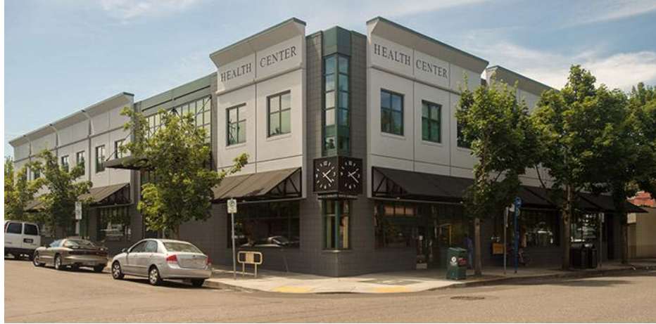
Multnomah County's North Portland Health Center recently received a $4.5 million renovation carried out by general contractor INLINE Commercial Construction . (Josh Kulla/DJC)
